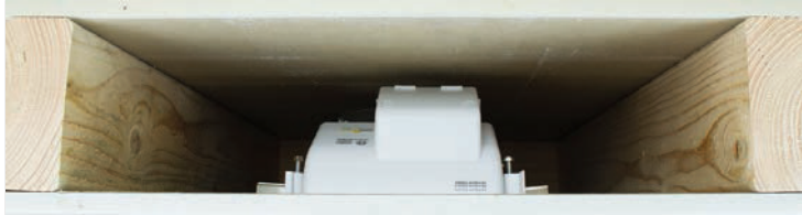
Figure 2: Cut out the supplied template on page 3 of this instruction sheet. Place the template on the wall in the desired install location. Using your pen or pencil, trace the template on the wall. Using a drywall saw or utility knife, cut a hole in the drywall the size of the template. See Figure 1 before tracing your opening. Remember, this wall plate is designed to be installed between the studs. It cannot be installed on top of a stud.
