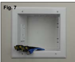
Figure 7: Your new Expandable Media Box with Duplex Surge Suppressor is now installed and ready for the TV mount to be installed. Install your TV mount bracket per the TV bracket manufacturer's instructions.
