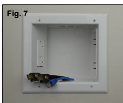
Figure 7: Your new Expandable Media Box with 20 Amp Duplex Receptacle is now installed and ready for the TV mount to be installed. Install your TV mount bracket per the TV bracket manufacturer's instructions.
