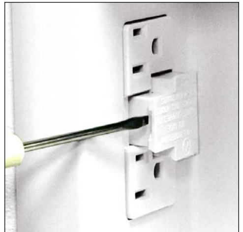
Removing the Surge Bloc® Module
